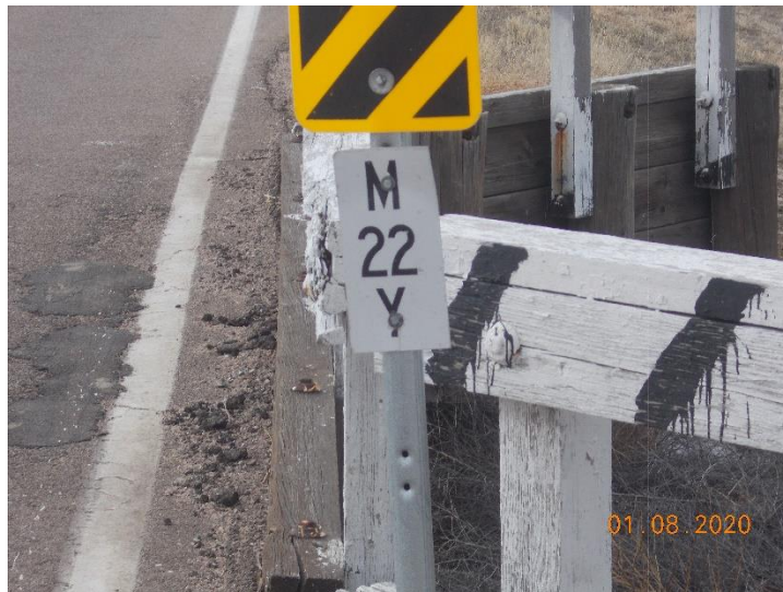
View of bridge M-22-Y signage.
