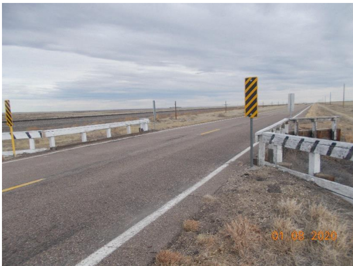
View of bridge M-22-Y looking northeast.
