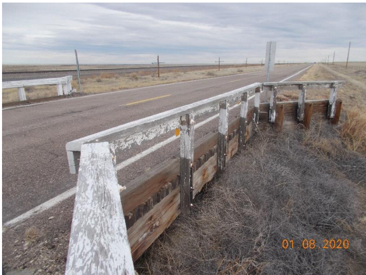
Side view of bridge M-22-Y.
